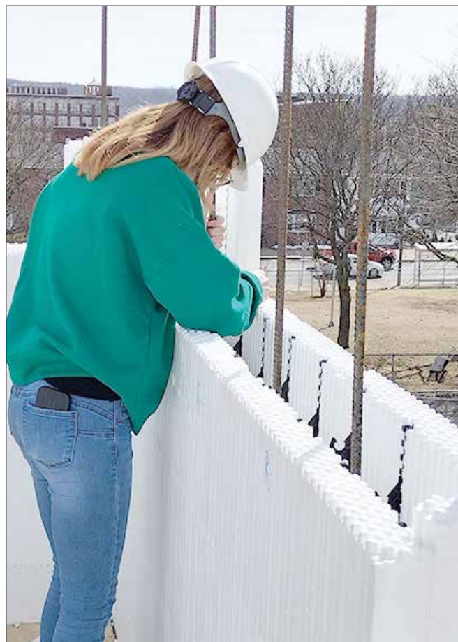
Dean student working with rebar at Chestnut.
