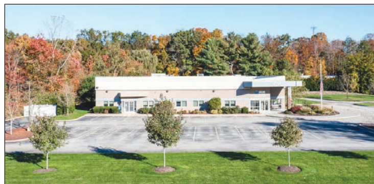
A cell tower can be installed at 1070 Suffield St., the site of the soon-to-be new Agawam Police headquarters once the council approves the second reading of the change to the wireless telecommunications overlay district.
