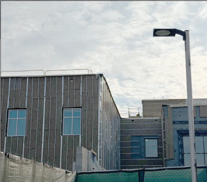
The first phase is brand new construction and should be ready near the end of 2026.
