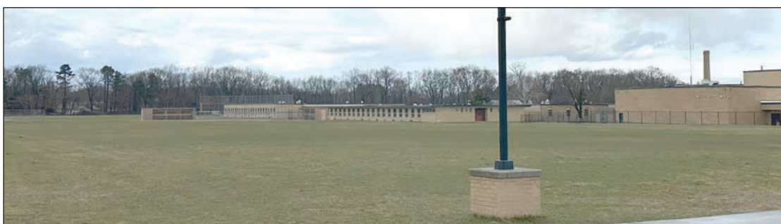
Construction would take place in phases with some new construction taking place next to the current building.
