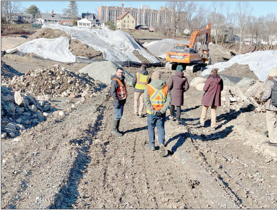
Construction is ongoing to restore Abbey Brook.
