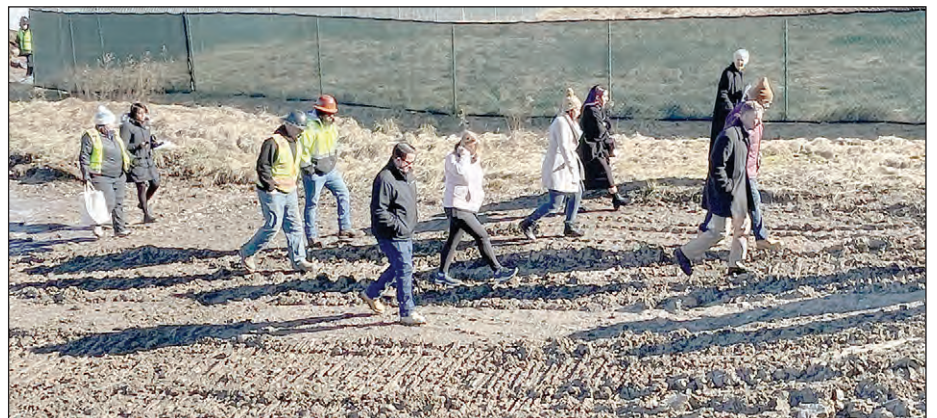
State and city officials toured the construction site in Szot Park on Tuesday.
