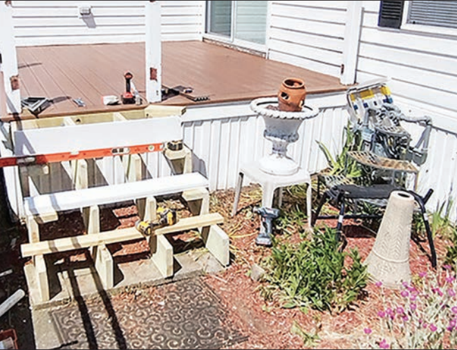
Wayne's new deck while it's under construction.
