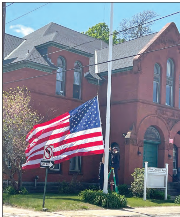
Crews raise the new flag up the pole at the senior center.
