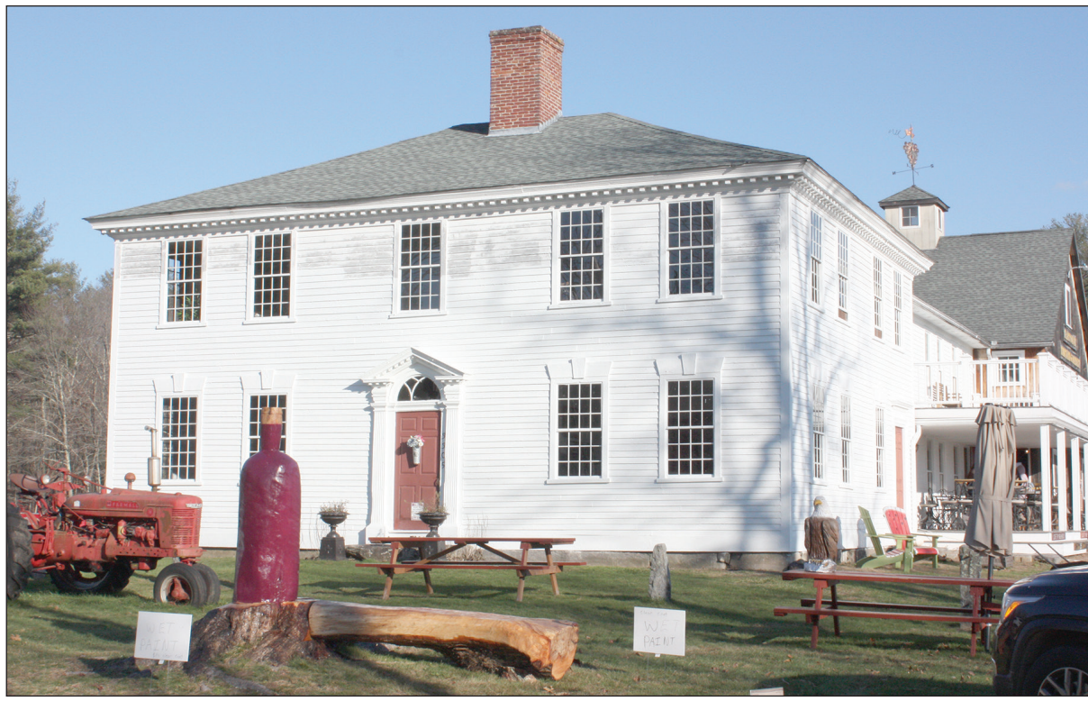
A view from the front of the winery shows off the majestic Federal-era, fully restored, mansion. The timber frame barn is on the back of the mansion, and is where the public comes to enjoy wine, food, and friends.
