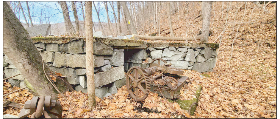
The site contains parts of equipment used for granite cutting and polishing
