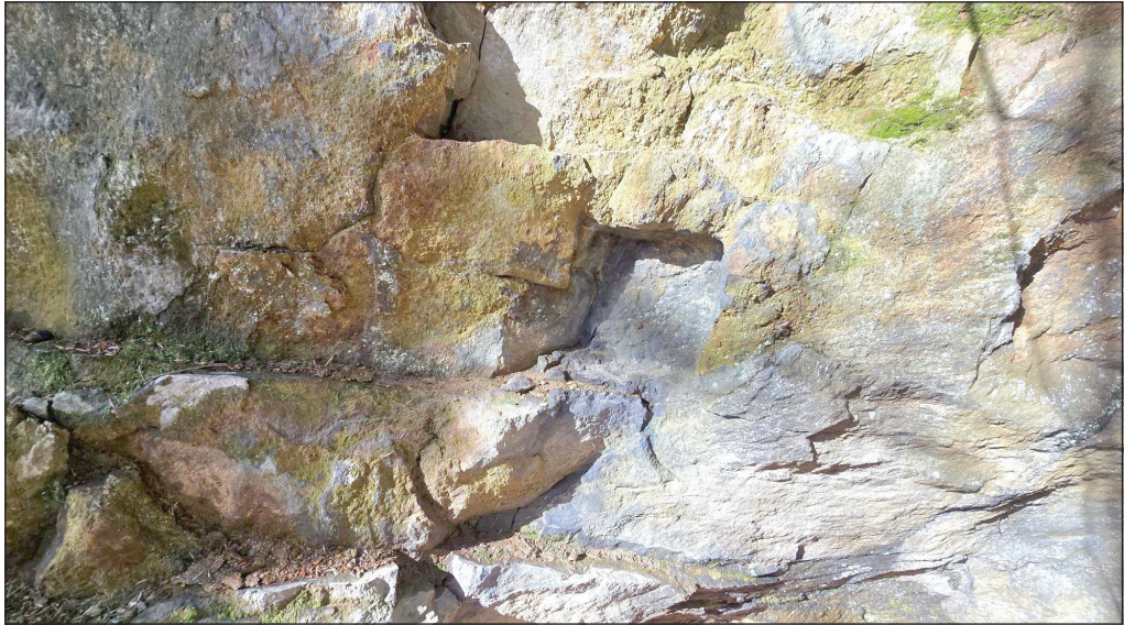
People can see the slot where a timber fit in to reinforce the mine shaft entrance.
