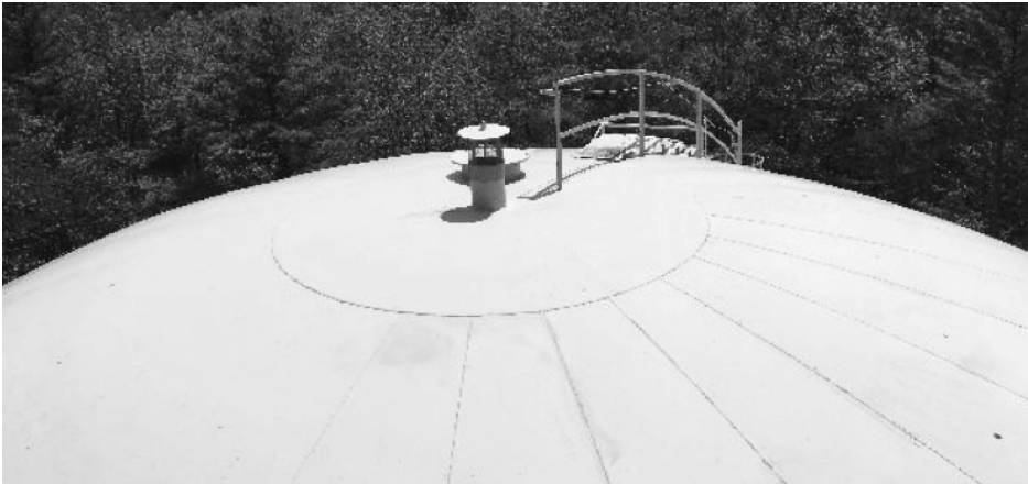
View from Anderson Road Water Tank Ware, MA
