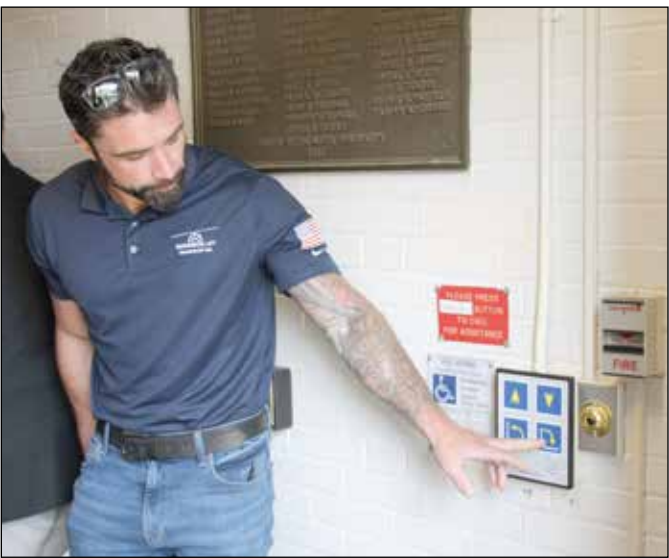
ABOVE: Adam Bishop of Garaventa Lift pointed to the chairlift’s wall control panel. LEFT: Town Administrator James Ferrera and resident Donald Neilsen are shown at the press conference announcing the installation of the new accessibility chairlift.
