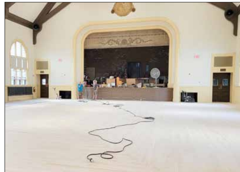
The floors to the main level of the Town Hall were sanded before being sealed.
