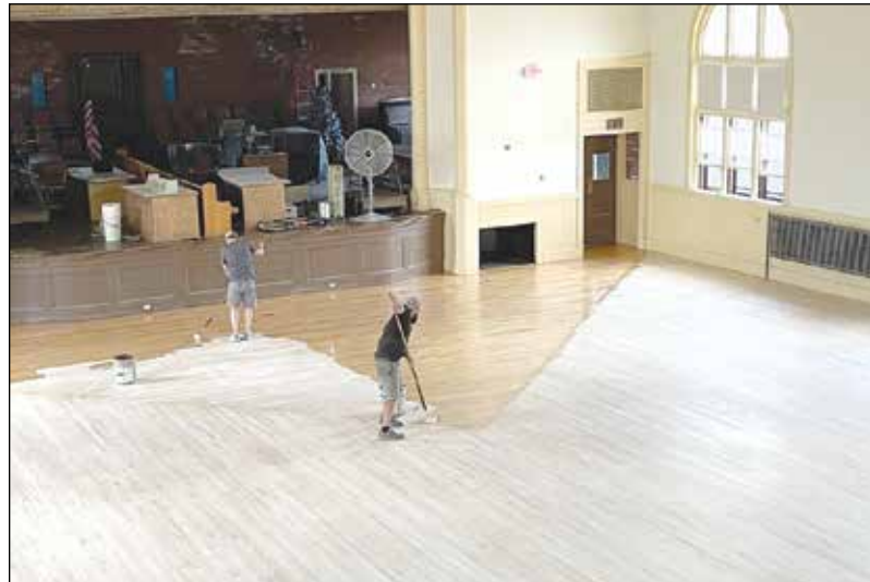
Workers apply the first coat of polyurethane.
