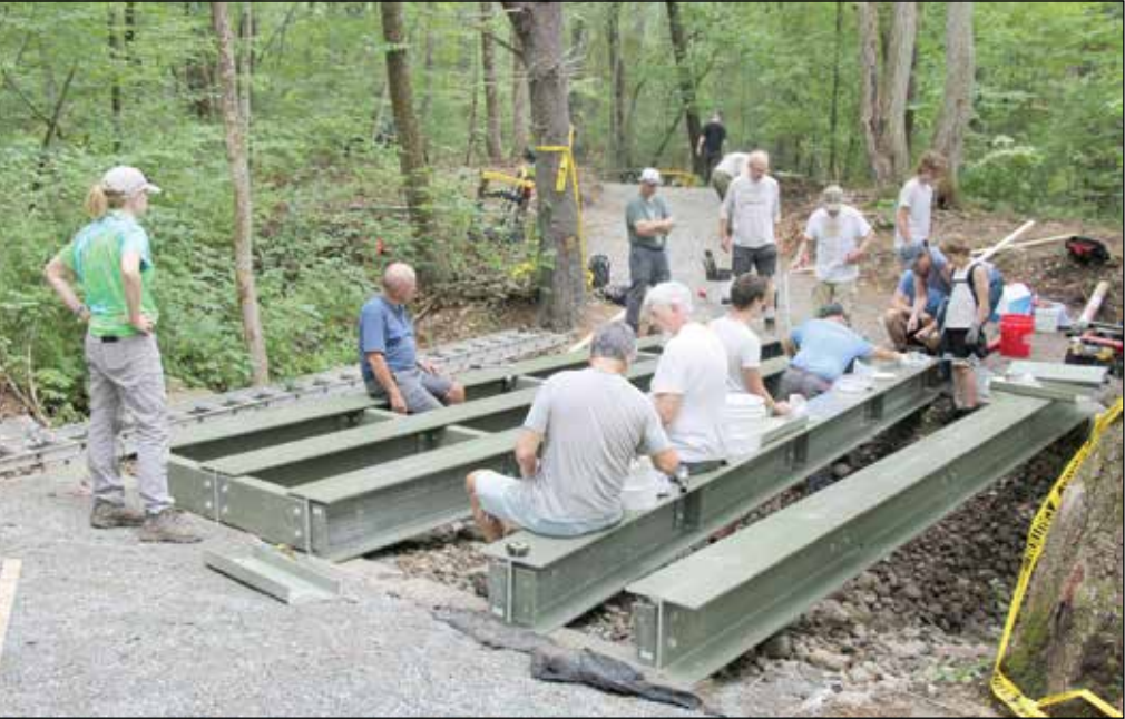
Volunteers worked to assemble the bridge on Aug. 21.
