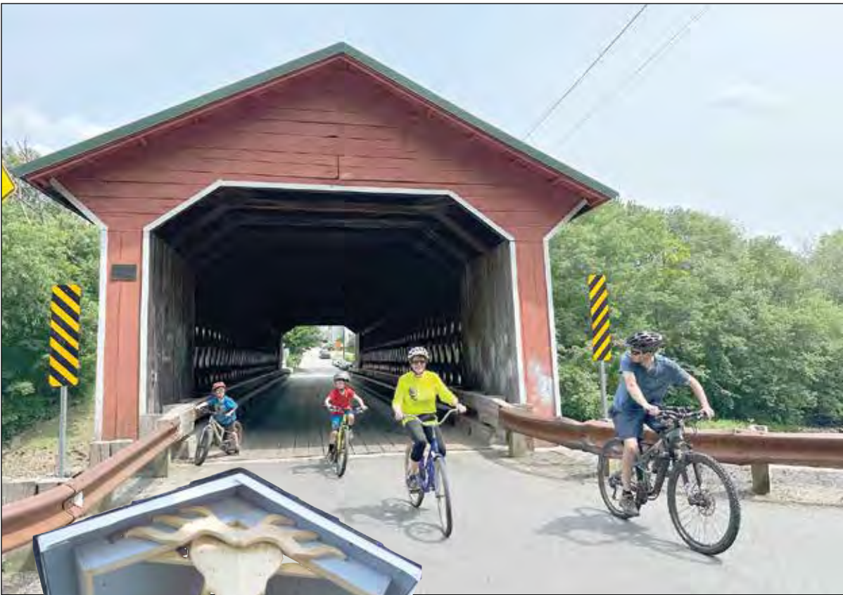
Trail users can cross from the gazebo at New Furnace Landing to the continuation of the rail trail, which leads to the Ware-Hardwick Covered Bridge.
