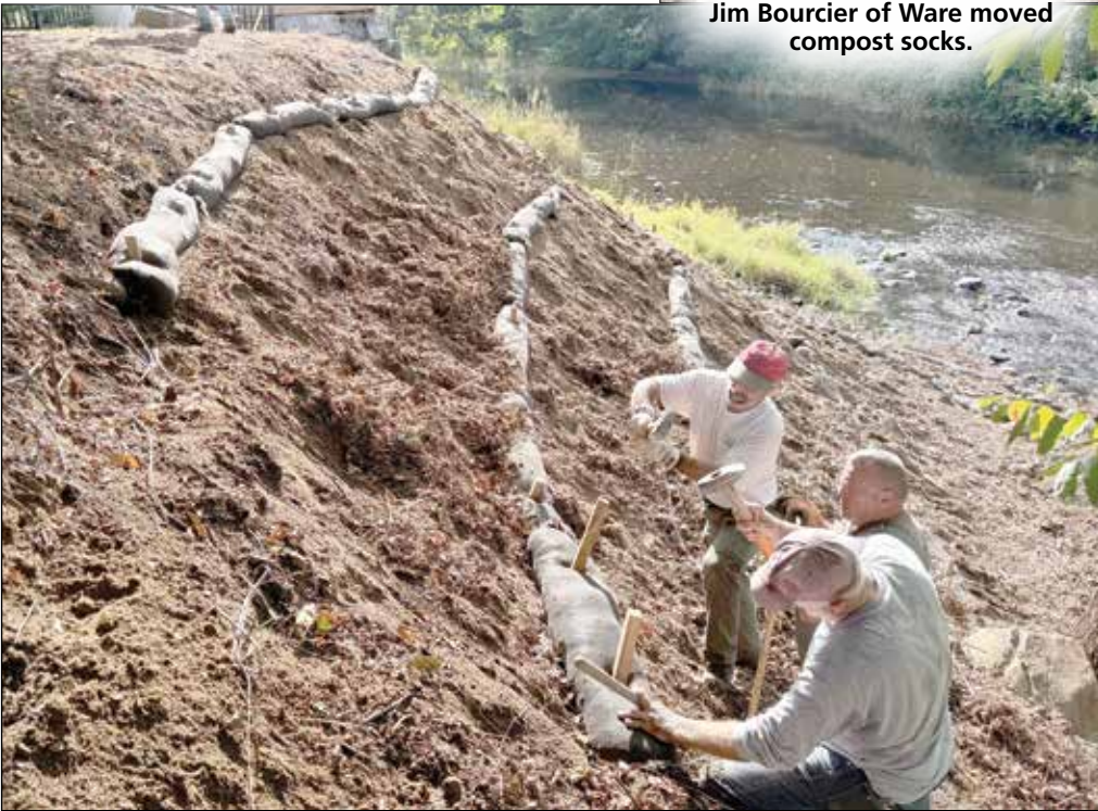
Compost socks are in place and ready for planting.
