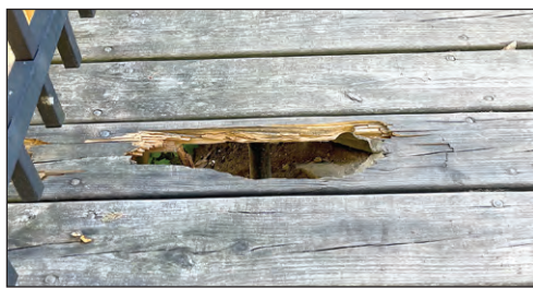
Rotten boards have been replaced on the walkway to the gazebo.
