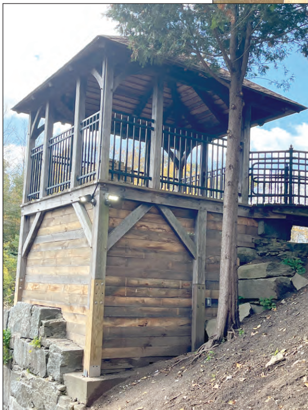
The underside of the gazebo was enclosed to protect it from vandalism and littering.
